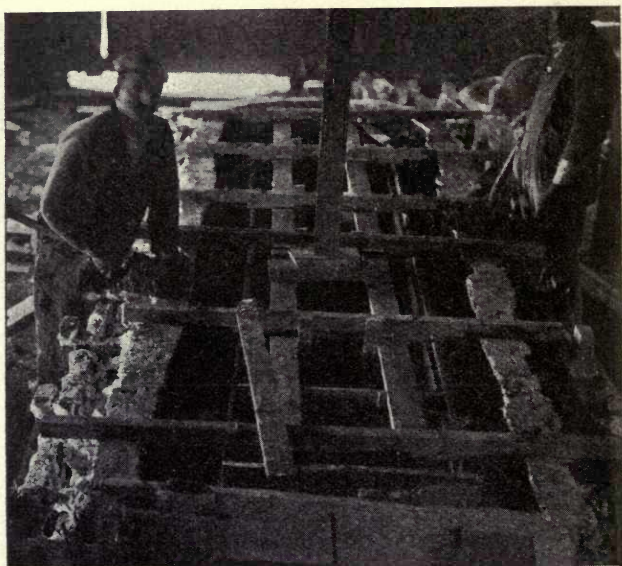
FIG. 46—FILLING PLASTER MOLD WITH CONCRETE. NOTE CORE TO MAKE STATUE HOLLOW
